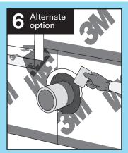
Alternatively, penetrations can be flashed with 3015UC after applying the field area membrane. Sealant should be applied to the top half of the 3015UC — field membrane transition to seal the negative lap.
